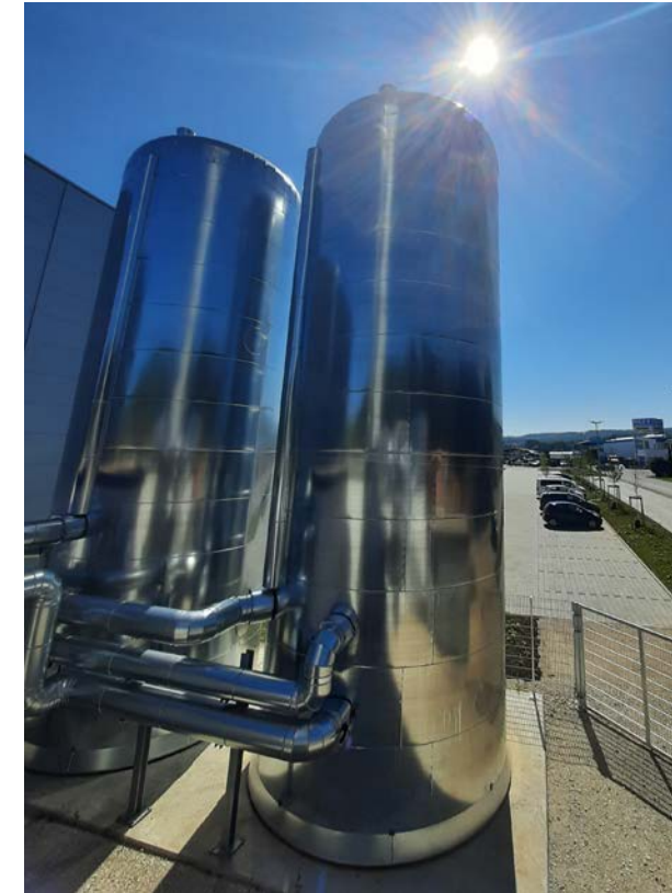
2 x 100 m 3 Pufferspeicher, Dettenhausen
